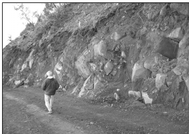
Figure 3. Cutting in talus slope
