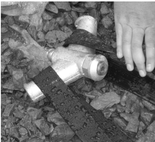
Figure 10. Connection of synthetic reinforcing strip to nail head.
