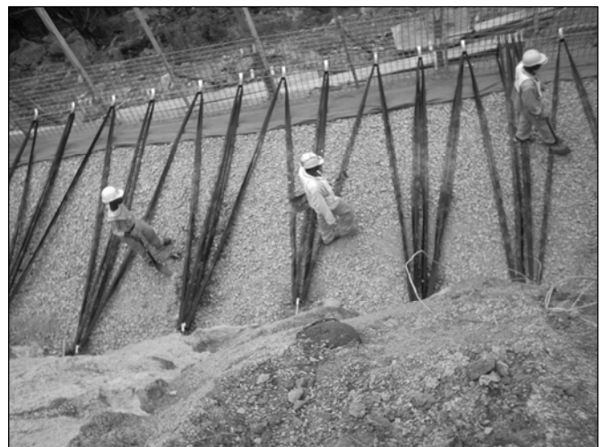
Figure 6. Placing of synthetic link reinforcement
