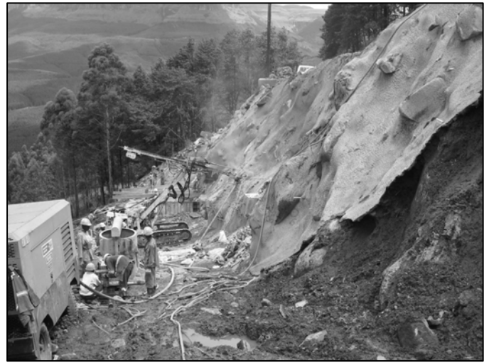
Figure 9. Installation of the soil nails
