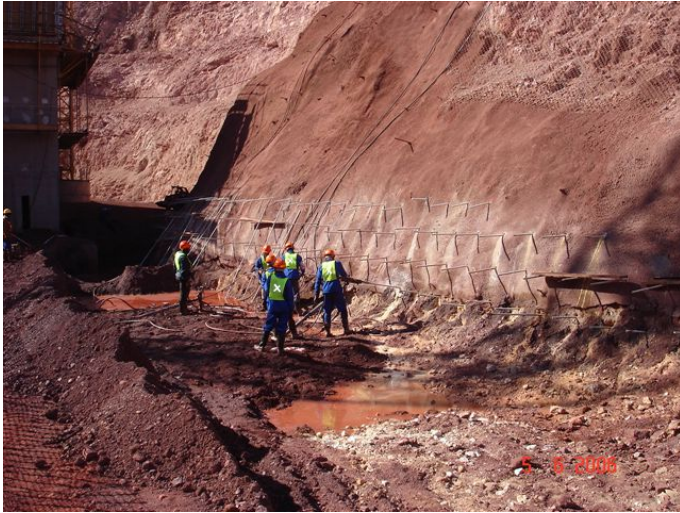
Figure 7. Nail installation
