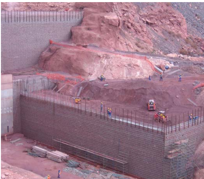
Figure 7. Wall B close to completion
