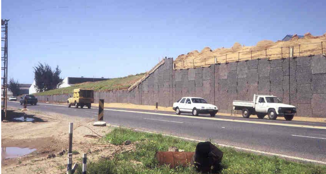
Figure 9. An abutment prior to construction of distribution beams
