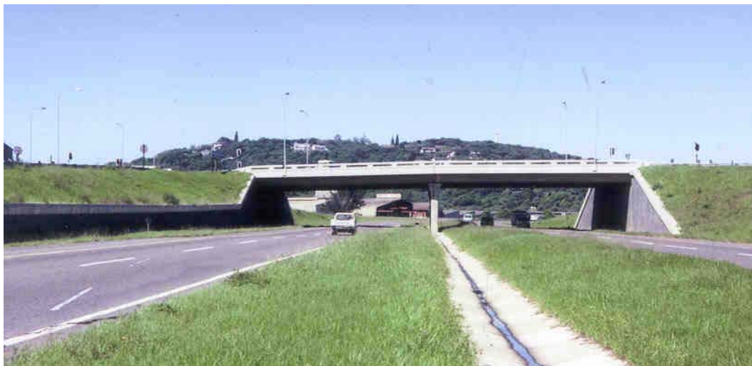
Figure 10. Completed bridge structure
